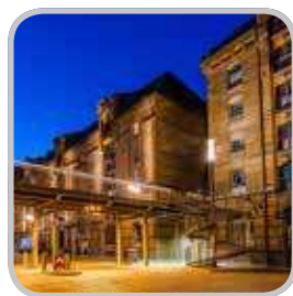
industriale industrial / industriel
